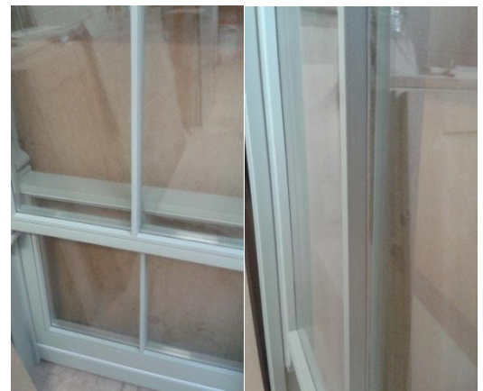
Vertical Stick on Beads without glazing parting beads
